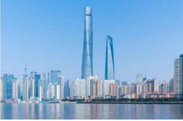
Shanghai Tower / China
