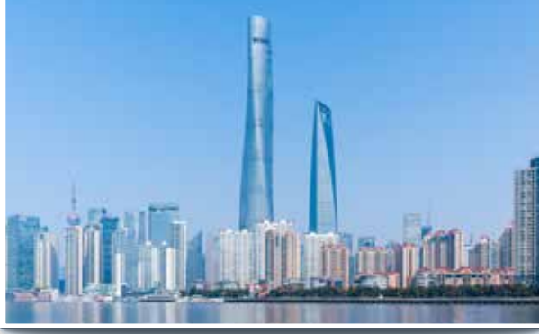
Shanghai Tower / China
